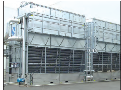
PCD Hood Installation
