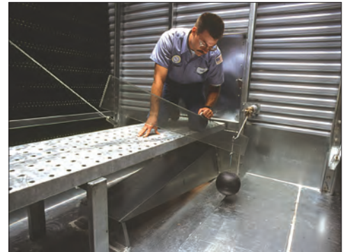
Mechanical Water Level Control
