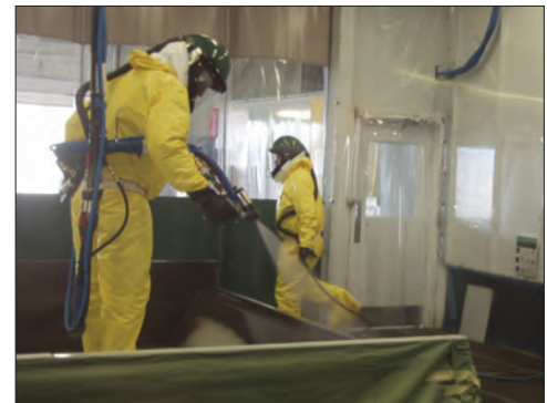
Application of TriArmor® Corrosion Protection System
